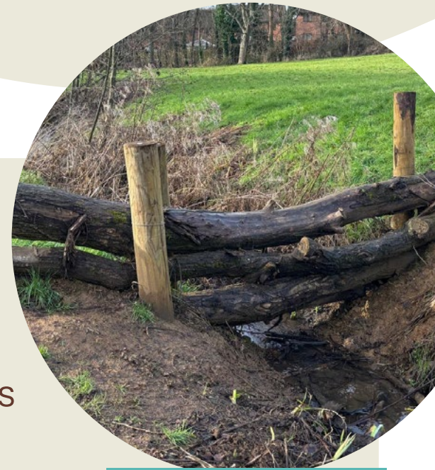
Example of leaky dam creating a natural barrier which slows the water flow, traps sediments, and minimises downstream flooding
